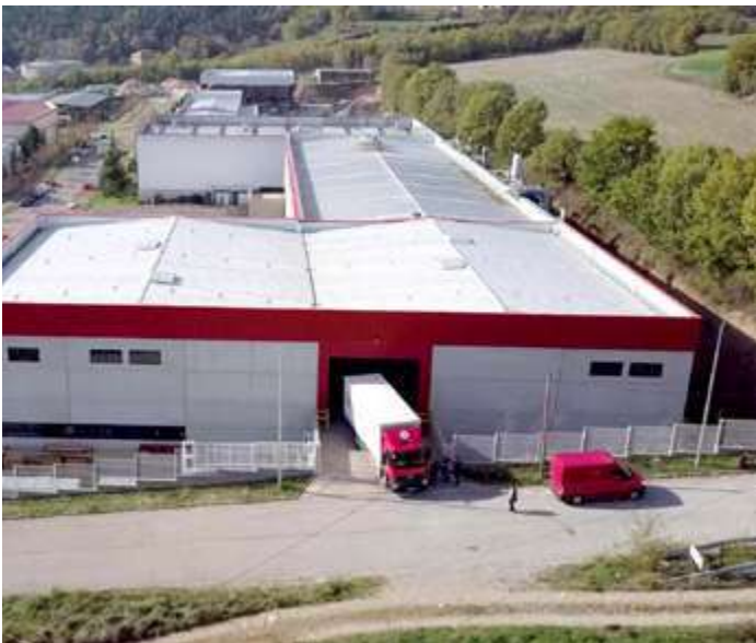
Technical textiles plant. Berga, Barcelona.
