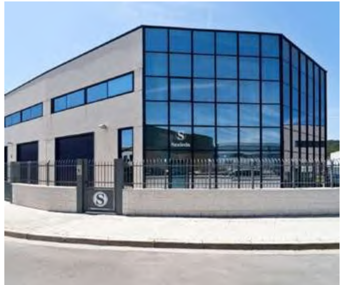
Logistic platform. Malgrat de Mar, Barcelona.
